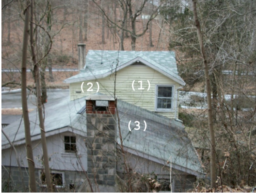
East Elevation View: (1) the second floor east bedroom with the original roofline above. (2) the 20th century bathroom addition with extended roof. (3) 20th century addition (family room and kitchen).
